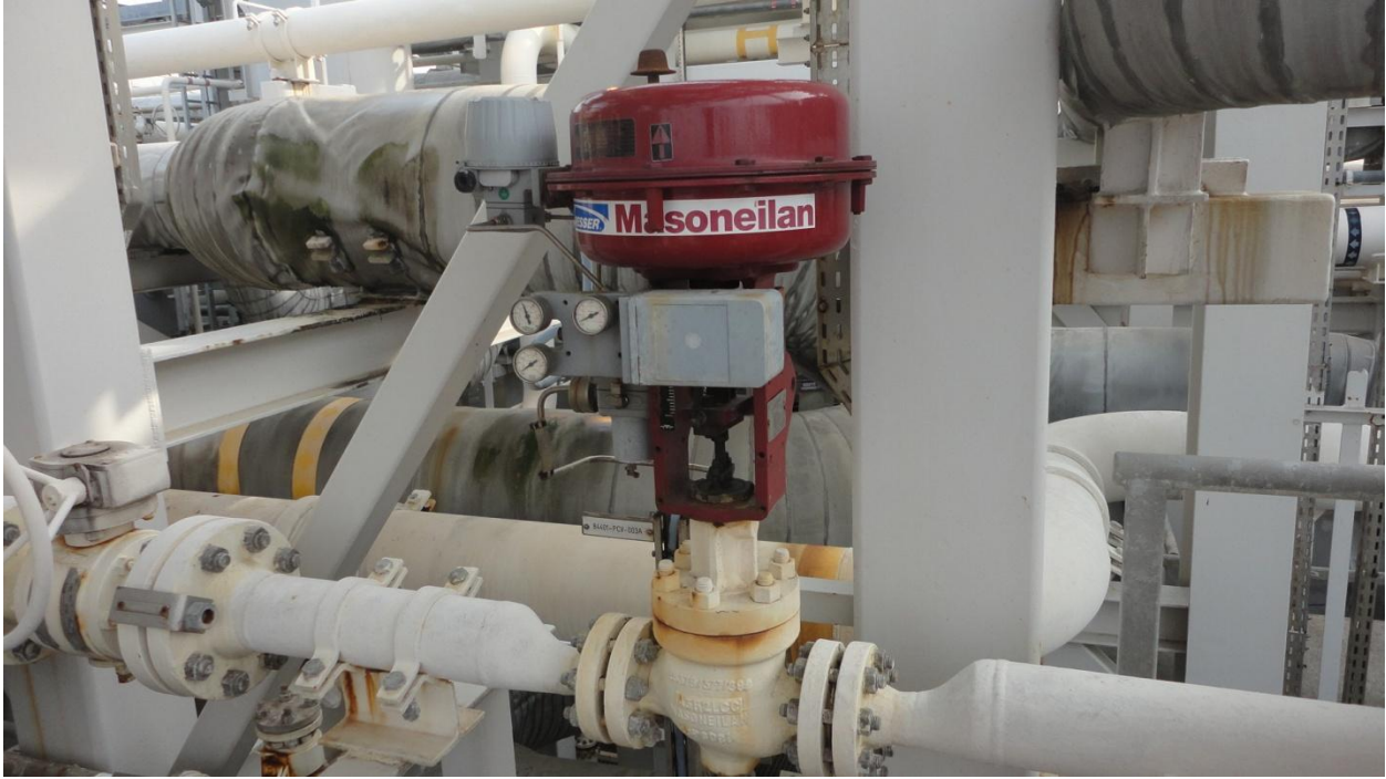
SPDC Equipment/ Control Room 6
