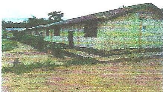
Classroom block constructed at Ichi, Ekwusigo L.G.A Anambra State
