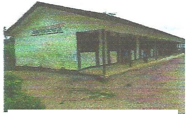
Classroom block constructed at Community Primary School Okpeze, Orumba North L.G.A Anambra State
