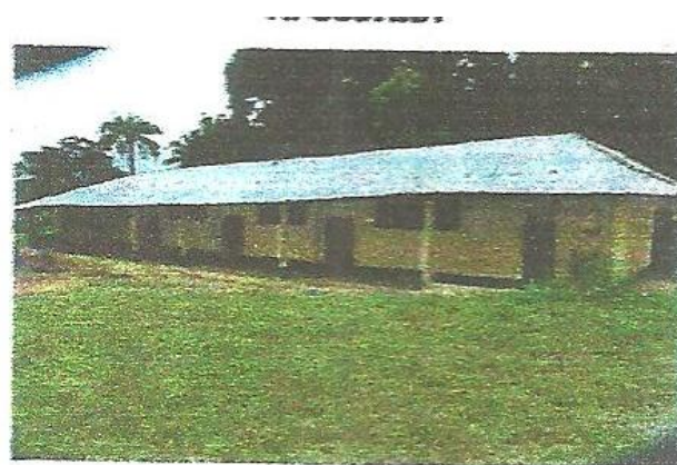
Renovated Classroom block at Okpoko, Ogbaru L.G.A Anambra State
