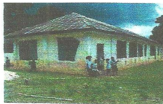
Renovated Classroom block at Ndiokpalaeze, Orumba North L.G.A
