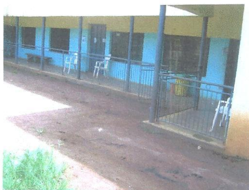
Health Centre constructed and donated to the Community at Akwaeze, Anaocha L.G.A Anambra State
