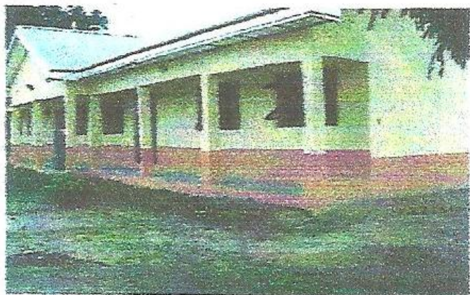
Classroom block constructed at Agulu, Anaocha L.G.A Anambra State
