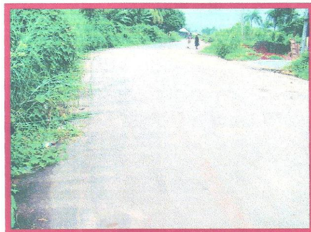
Road rehabilitated by Age Grade in Ufuma
