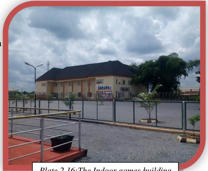
Plate 2.16: The Indoor games building at Awka wonderland. Source: Researcher's Survey (2016)
