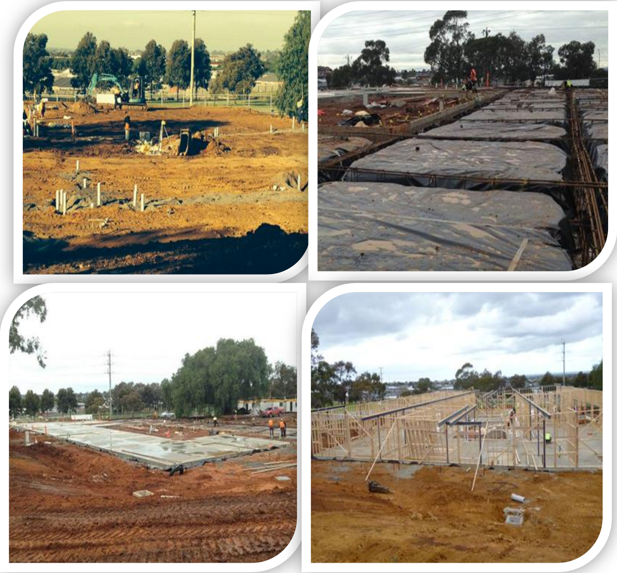
Plate 2.43: Goodstart Waurm Ponds at various stages of construction / Source: Goodstart media (2016)
