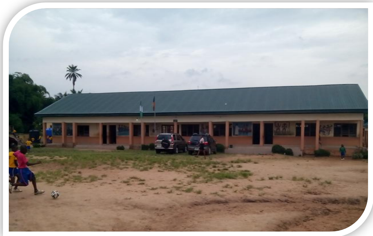
Plate 2.11: front elevation of a classroom | Source: Researcher's survey (2016)
