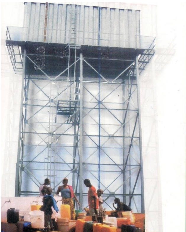
Comprehensive Water Project, Initiated and Completed by Hon. Jaunty Okwudi Administration and Commissioned by the Deputy Governor of Delta state, His Excellency, Prof. Amos Utuama, June 2010.
