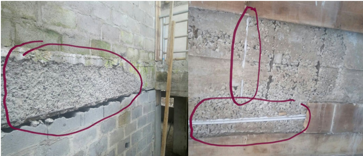
Plate I: An exposed reinforcement bar in Plate II: Collapsed yet-to-be completed road a raking floor beam (Sources: Researchers Field Work, 2018 )
