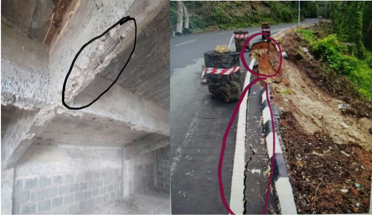
Plate I: An exposed reinforcement bar in Plate II: Collapsed yet-to-be completed road a raking floor beam (Sources: Researchers Field Work, 2018 )
