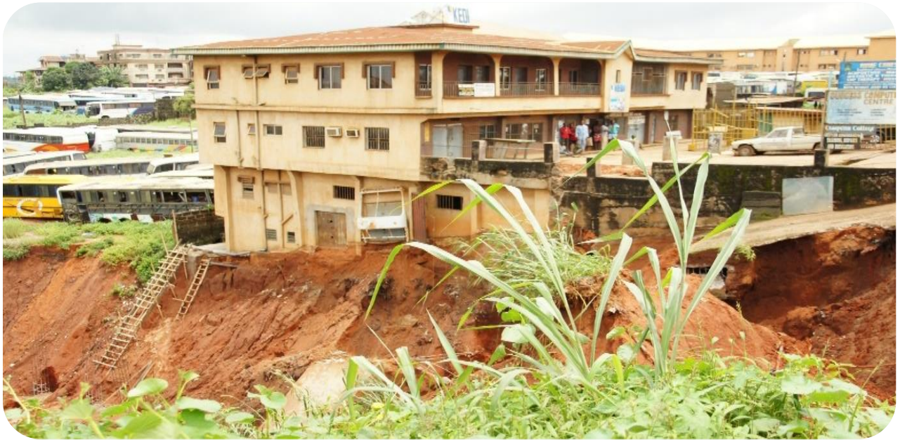
Fig. 4.16 New Heritage Omagba/Onitsha Erosion Site, 2013 before NEWMAP
