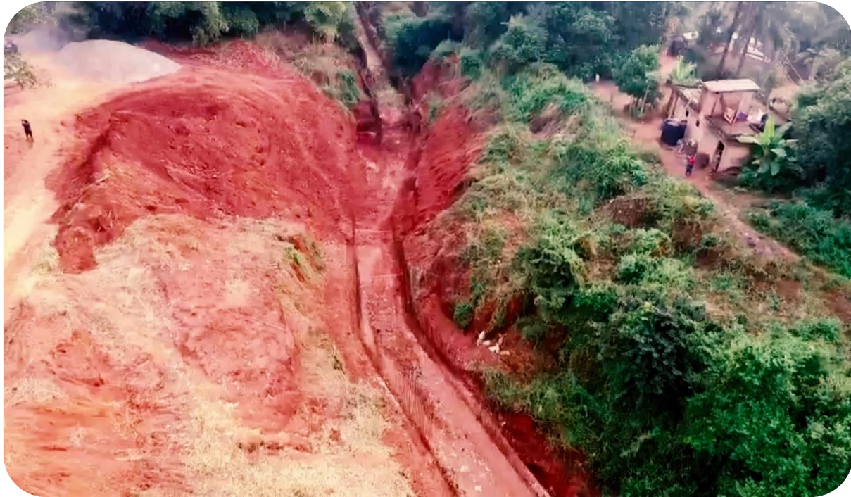
Fig. 4.12 Abagana Erosion Site, 2013 Before NEWMAP Intervention
