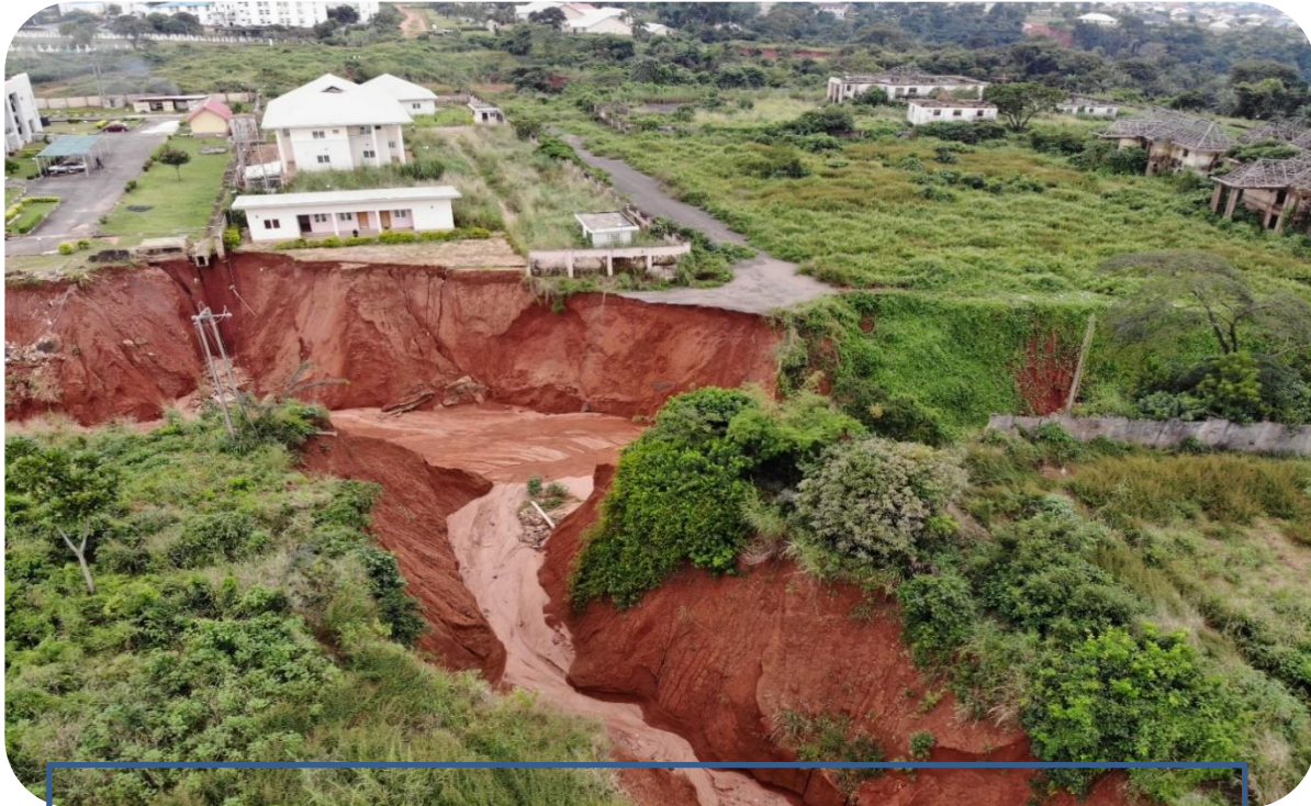
Fig. 4.20 Ekwueme Square/Fed. High Court Erosion Site, 2013 Before Phase I NEWMAP
