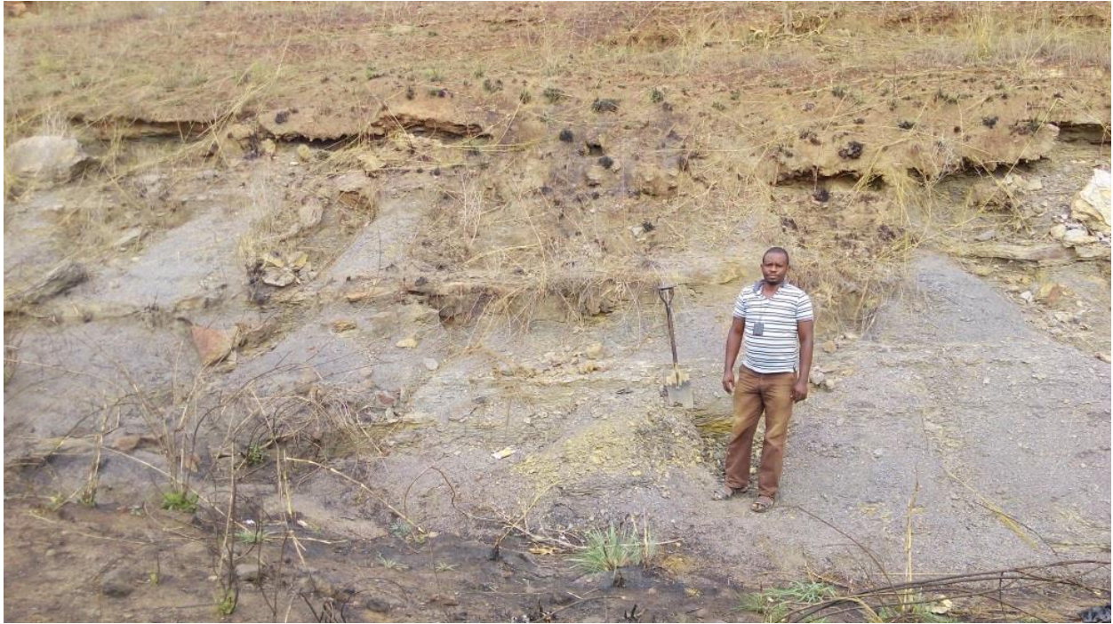
Fig. 4.18b: Photograph of the Outcrop Section at Akagbe-Ugwu, along Port Harcourt to Enugu Exp. Way, Enugu State.
