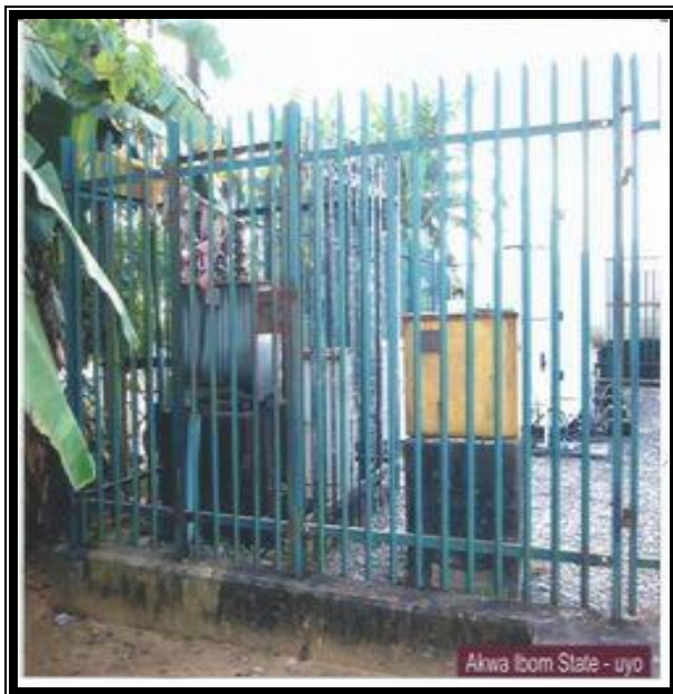
Figure 6: Etukapan Quarters, Etan compound (3 Meters to the house, 35 meters in height)
