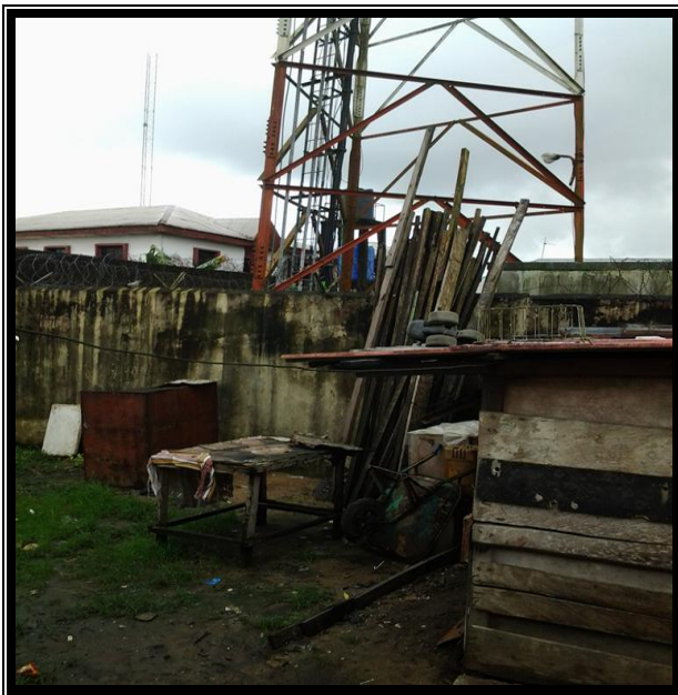
Figure 12: Amarata Quarters; Tamarakero Compound 1 meter to houses, 30 meter in height
