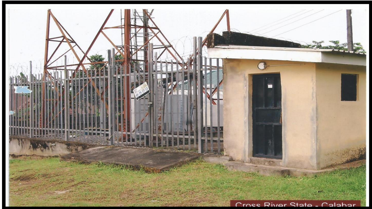
Figure 16: Sabongari Quarters; Edet Compound (2 meters to houses, 35 meters height)
