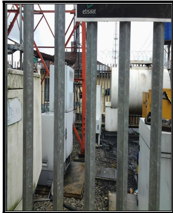
Figure 35: Rumukoro Quarters; Wikimor's compound (1meter to the house, 20 meters in height)
