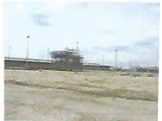
Stacking Area (4,216.80m 2 )
