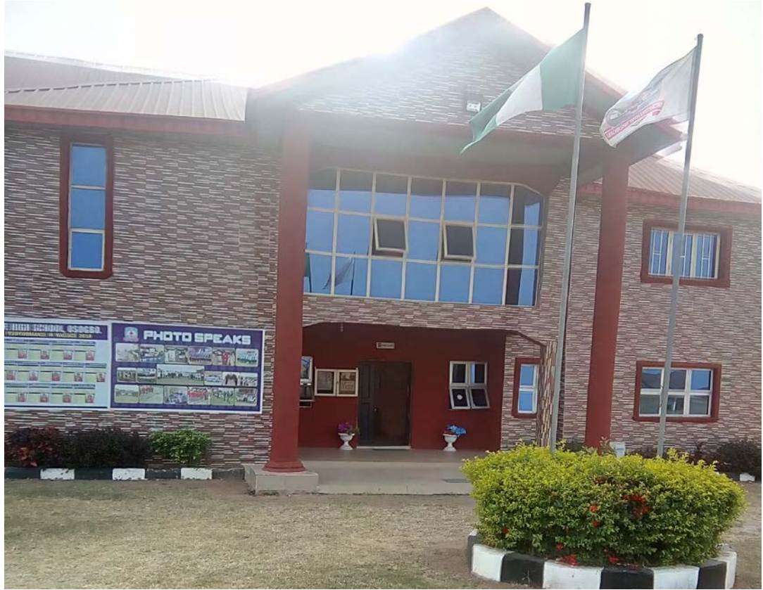
Plate 11: Picture Showing DLHS Osun State Administrative Block
