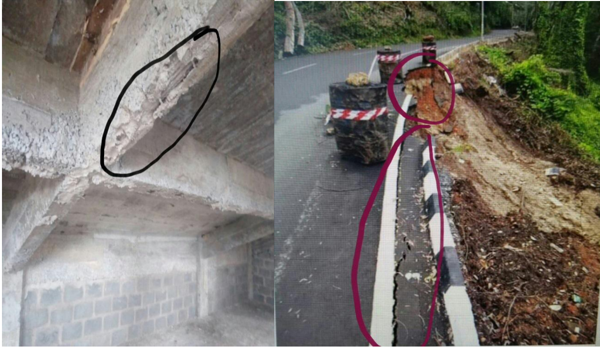
Plate I: An exposed reinforcement bar in a raking floor beam Plate II: Collapsed yet-to-be completed road (Sources: Researchers Field Work, 2018)
