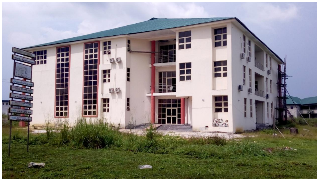
Department of Music building Uniport near completion
