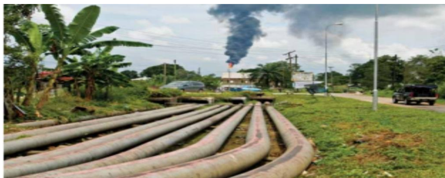
Figure 3: Exposed pipelines flaring gases traversing community in Niger Delta
