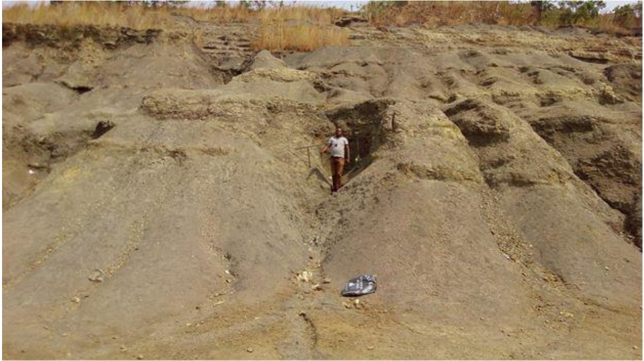
Fig. 4.24b: Photograph of the Outcrop Section at Aluson Petrol Station, along Enugu to Onitsha Exp. Way, Enugu State
