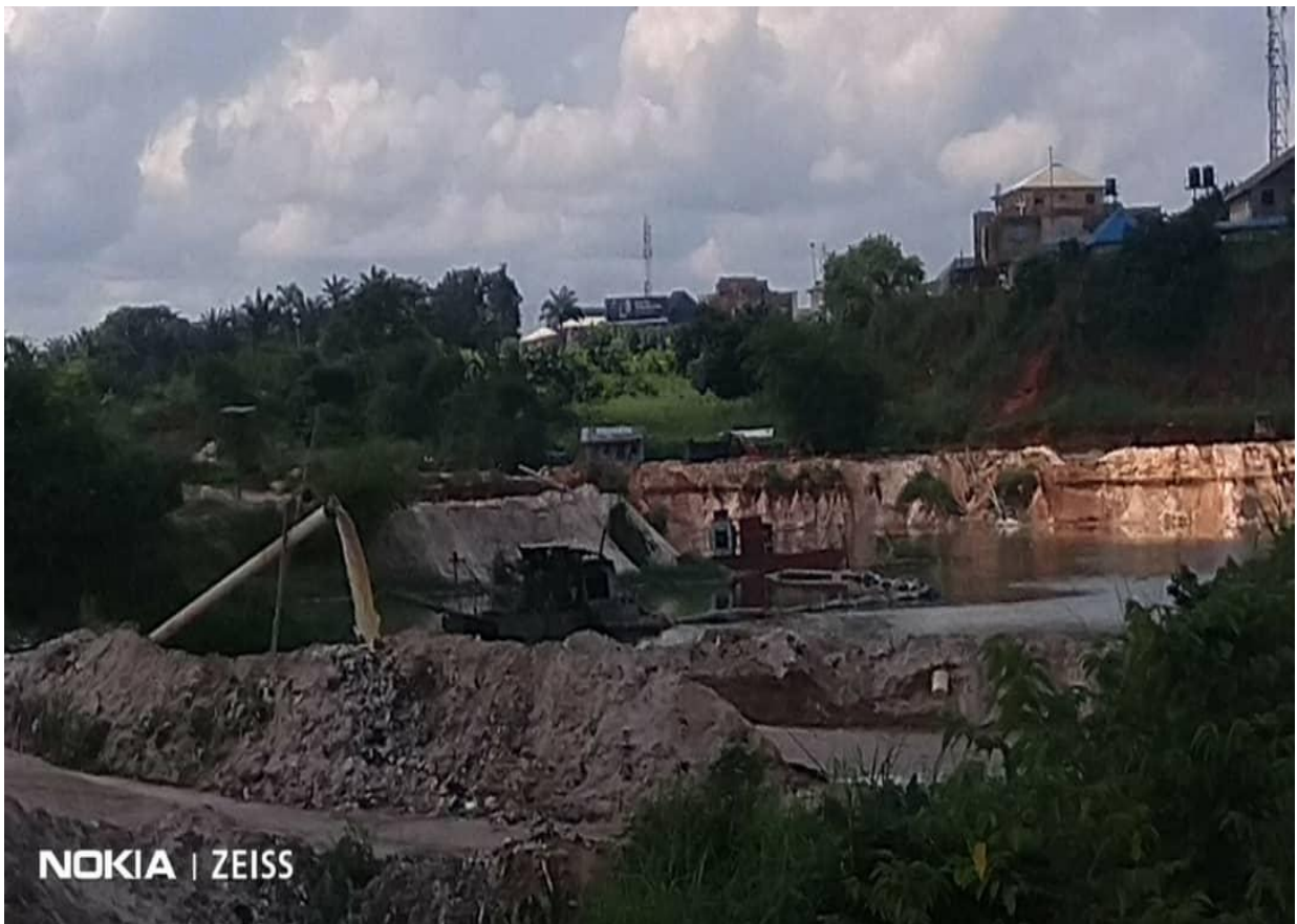
Plate i. Sand Mining/Dredging in Otamiri River, adjacent Mechanic Village, Nekede
