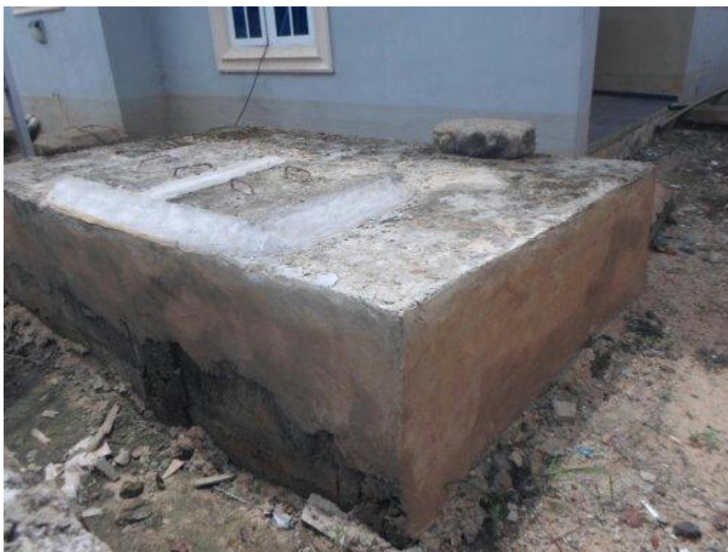
Plate 5.12 A Soakaway Pit previously covered by flood water
