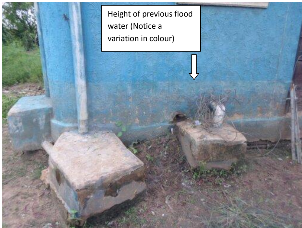
Plate 5.11 A Previously Covered Soakaway Chamber
