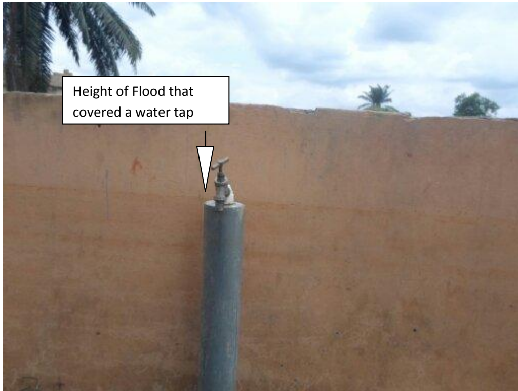
Plate 5.14 A Previously Covered Source of Pipe borne Water
