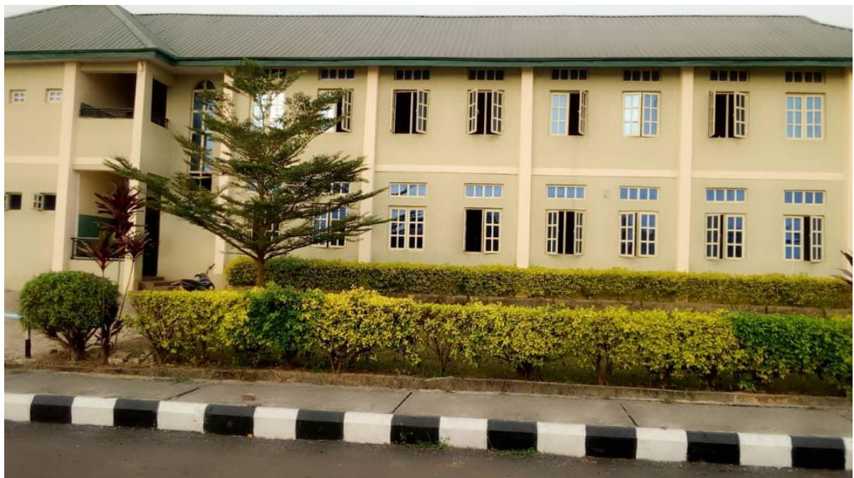
Plate 10: DLHS Akure Multi-purpose Block
