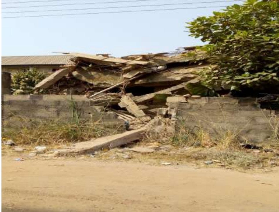
Plate 5.7: Building collapse in the study area
