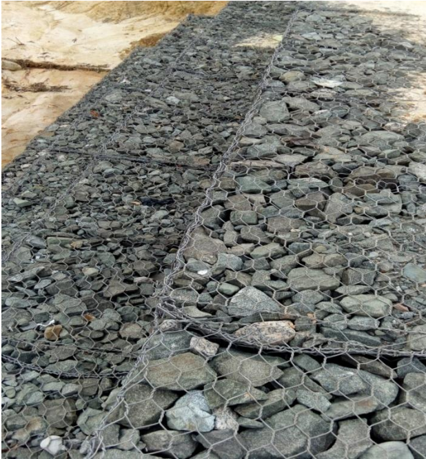
2a. Gabions after construction by Rhino at Nanka Erosion Site (Researcher's Field Work Pictures)
