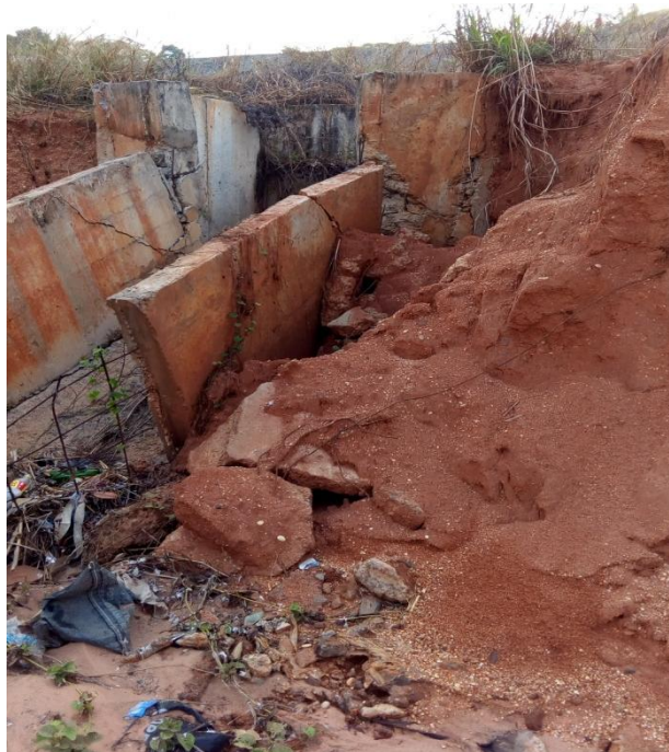
2g. Failed Gully Erosion Channelization at Neni
