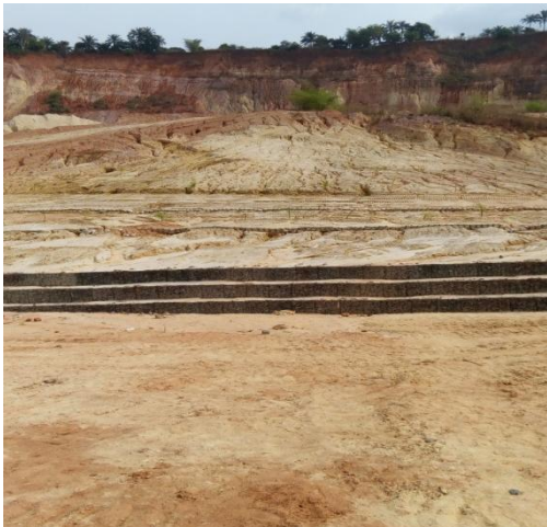
2c. Gabions showing signs of failure a short while after construction at Nanka Erosion Site (Researcher's Field Work)
