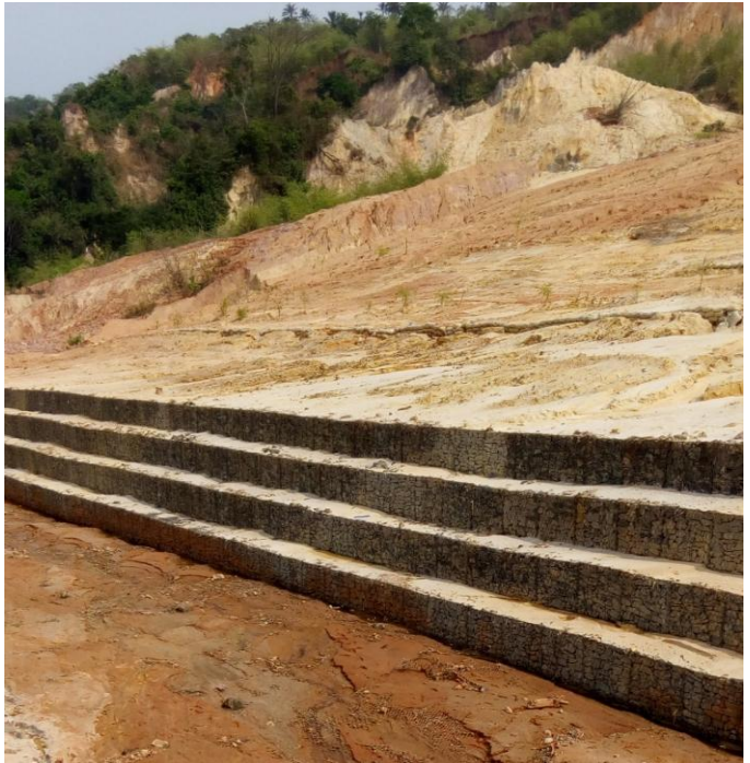
2b. Gabions after construction by Rhino at Nanka Erosion Site (Researcher's Field Work Pictures)
