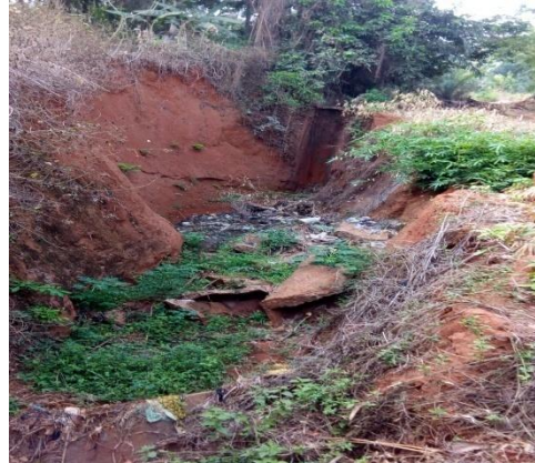
2f. Failed Gully Erosion Channelization at Oraukwu
