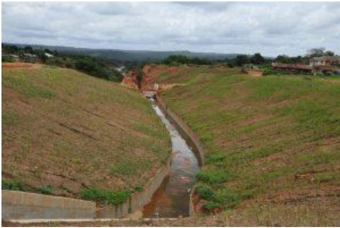
1e. Civil works mixed with bioremediation in one of the Auchi Gully fingers reclaimed by NEWMAP
