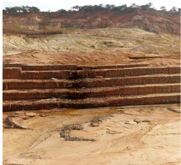
2d. Sandbag Check Dams showing signs of failure shortly after construction by Rhino at Nanka Erosion Site (Researcher's Field Work)
