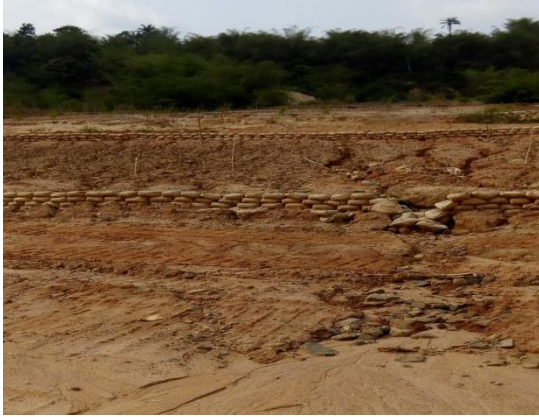
2e. Sandbag Check Dams showing signs of failure shortly after construction by Rhino at Nanka Erosion Site (Researcher's Field Work)
