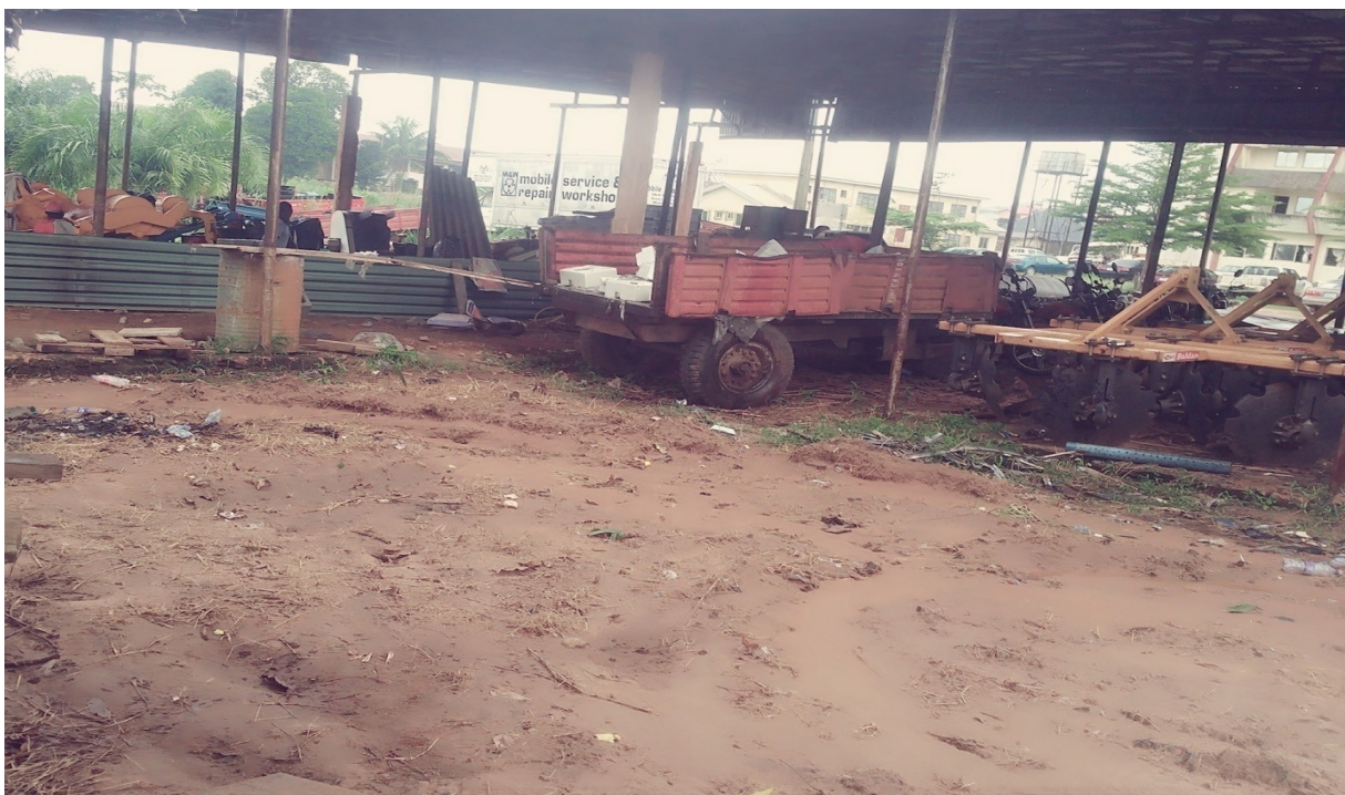
PLATE 2: Open shed implement shelter at the Anambra State agricultural ministry headquarters, Awka Nigeria
