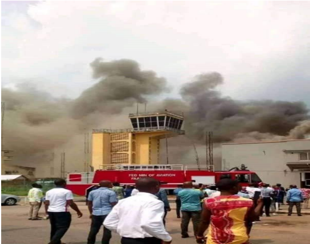
Plate: A13Arrival Section of Imo Airport gutted by Fire. Source: The Nation , April 9, 2019.
