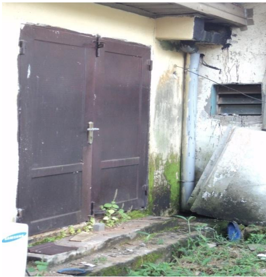
Plate 27: leakage of Concrete Slab and stains at the wall of CHER building at NAUTH, Nnewi
