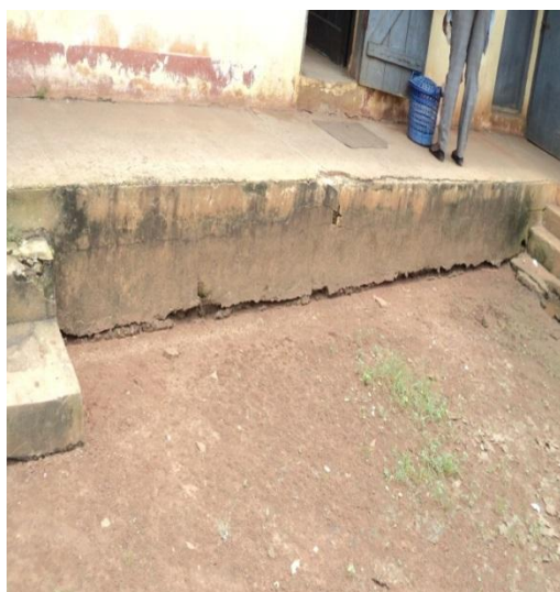
Plate 67: Horizontal Cracks caused by Stagnated water at dietetic building at NAUTH, Nnewi.
