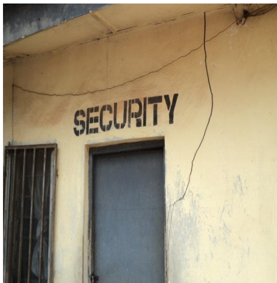
Plate 23: Vertical/Horizontal Crack at the security gate at NAUTH, Nnewi.
