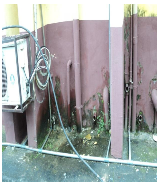
Plate39: Leaking Sanitary Pipes at the Laboratory Complex, at NAUTH,Nnewi. Source: Researcher's field study (2017)
