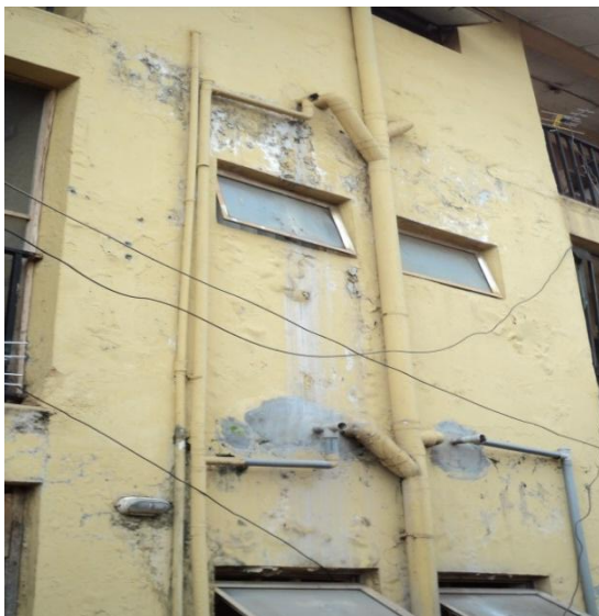
Plate 31: Flaking of paint walls at the walls of Doctors Call building at NAUTH, Nnewi
