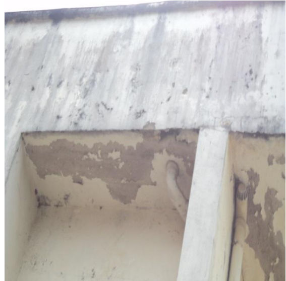
Plate 28: Leakage of concrete slab at Gutter of the radiology building at NAUTH, Nnewi.
