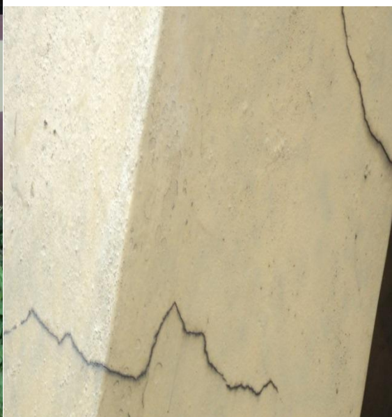
Plate 56: Cracks at the external walls of the VAMED block at NAUTH,Nnewi.
