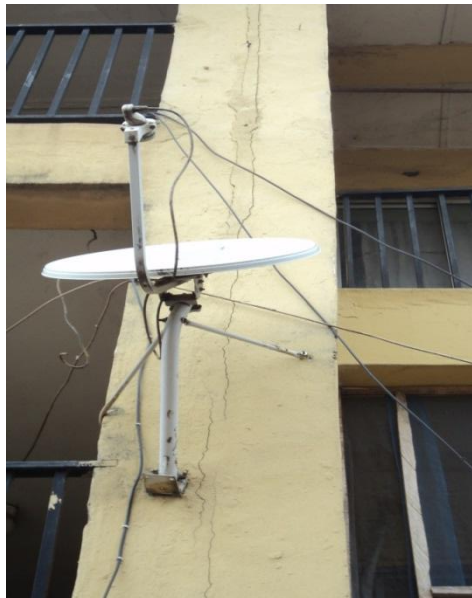
Plate 63: Vertical Cracks on walls at the ward Complex at the NAUTH Truma centre, Oba
