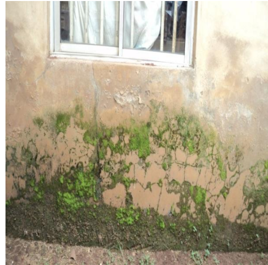
plate 6: Cracked walls caused by efflorescence at Back of GOPD, NAUTH, Nnewi. source: Researcher's field study (2017)
