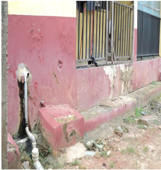
Plate 61: Defects, Flake and stains on external Walls of the quarters at NAUH CHC Ukpoko
