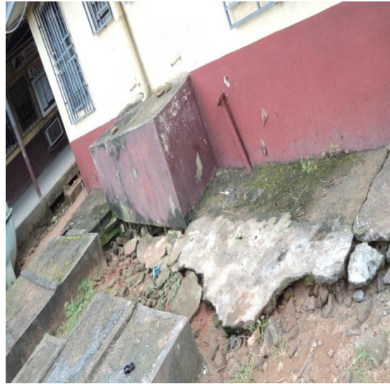
Plate 10: Defective Concrete Pavement Floor at the Corper Lodge, CHC, NAUTH Ukpo
