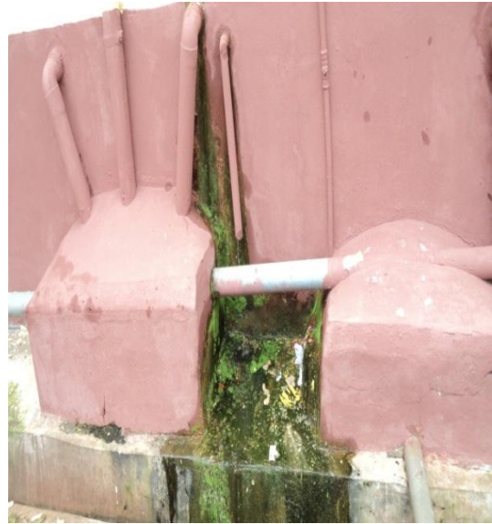
Plate 30: Efflorescence caused by dampness and leakage of pipes at the back of medical Complex, at NAUTH CHC Neni .
