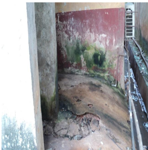
Plate 45: showing Moisture effect on walls/floor Of the Clinic at NAUTH CHC Neni. Source: Researcher's field study (2017)
