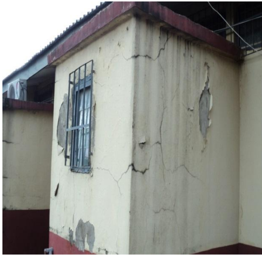
Plate 17: Diagonal Crack discovered on the External Wall of HIV-Lab at NAUTH CHC Ukpo
