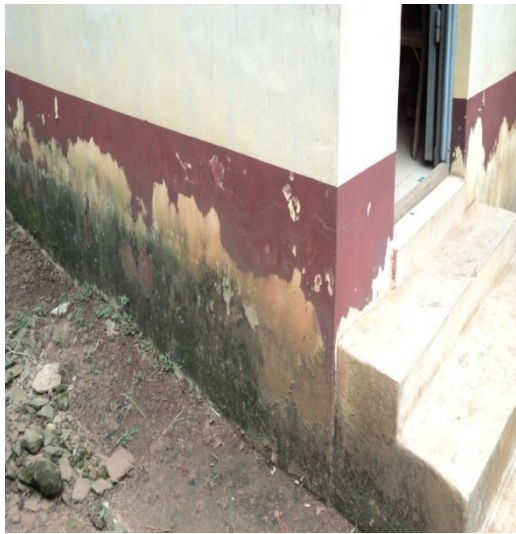
Plate 29: Flaking of Paint wall at the maternity Building, NAUTH, Awka
