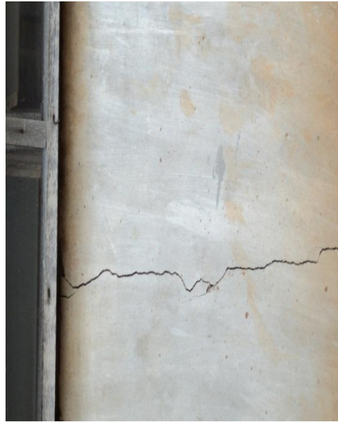
Plate 42: Vertical Cracks at the front of the SON Building at NAUTH,Nnewi. Source: Researcher's field study (2017)
