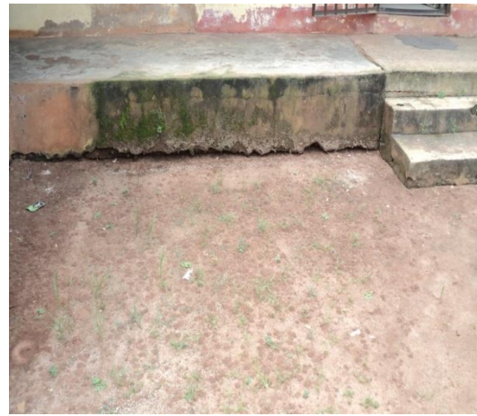
Plate 2: showing Crack and Dampness at the Foundation level of PCR Block at NAUTH Nnewi.
