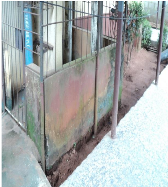
Plate 35: Efflorescence stains at the gas dump at NAUTH, Nnewi. Source: Researcher's field study (2017)
