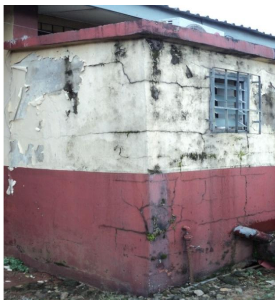
Plate 68: Multiply vertical/horizontal cracks and stains caused by water leakages in the public Toilet at NAUTH , Nnewi
