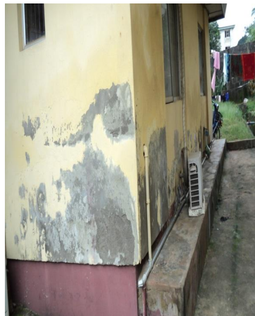
Plate 64: Defects/ Flaking of paint at the external wall of the Main building at the NAUTH CHC Neni
