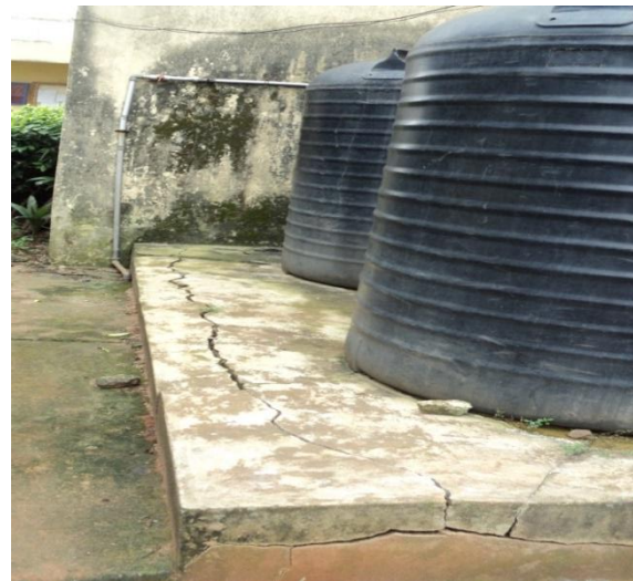
Plate 12: Crack found at the Floor of the pharmacy Building at NAUTH,Nnewi
