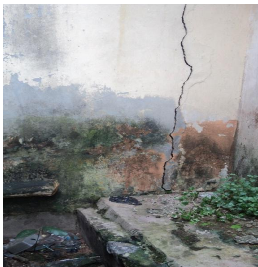
Plate 3: Crack and Dampness at the Foundation Level of Female Surgical Ward at NAUTH Nnewi
