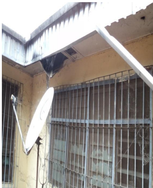
Plate 59: Falling/Bulging of ceiling boards at the back of the female surgical ward at NAUTH Nnewi.
