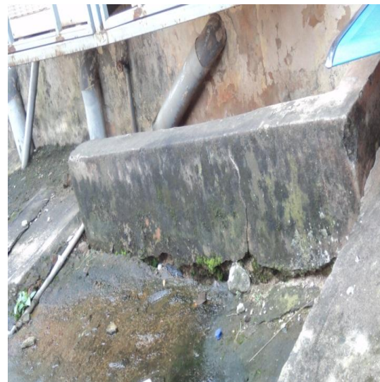
Plate 3: Crack and Dampness at the Foundation Level of Female Surgical Ward at NAUTH Nnewi
