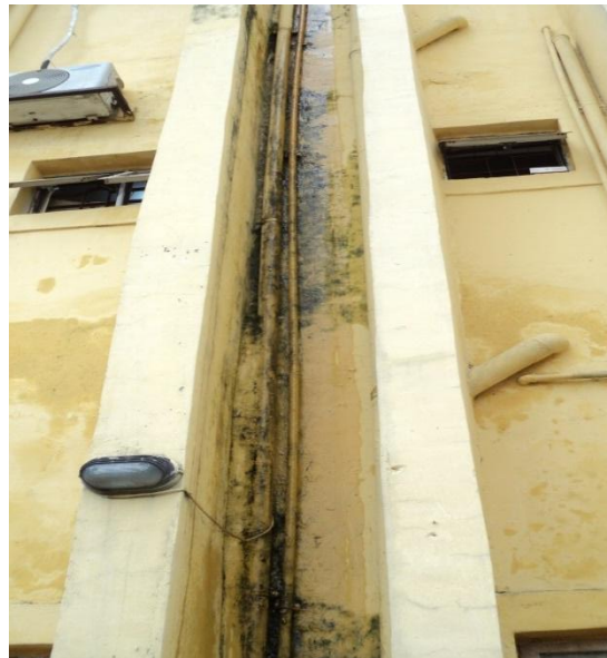
Plate 44: Leaking plumbing Pipes at the back of the Ward of NAUTH GEC Onitsha. Source: Researcher's field study (2017)
