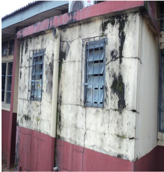
Plate 5: Longitudinal, Vertical and Diagonal Cracks/Dampness at Administrative block at NAUTH, Nnewi Source: Researcher's field study (2017)
