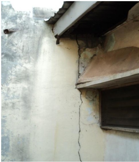
Plate 41: Defective and cracks walls at the Back of the SON building at NAUTH,Nnewi. Source: Researcher's field study (2017)
