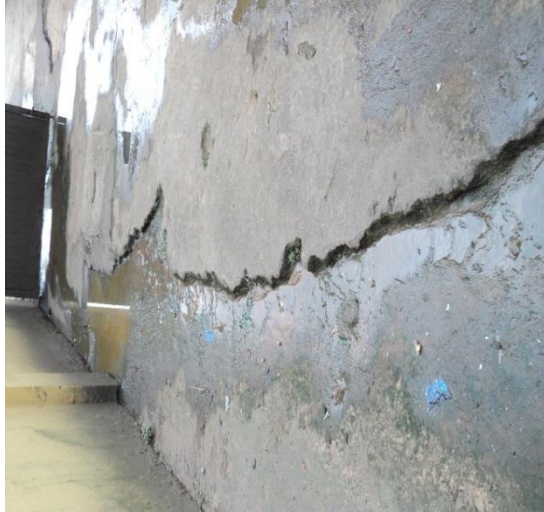
Plate 7: Cracked Floor slab at laboratory Complex at NAUTH Nnewi Source: Researcher's field study (2017)
