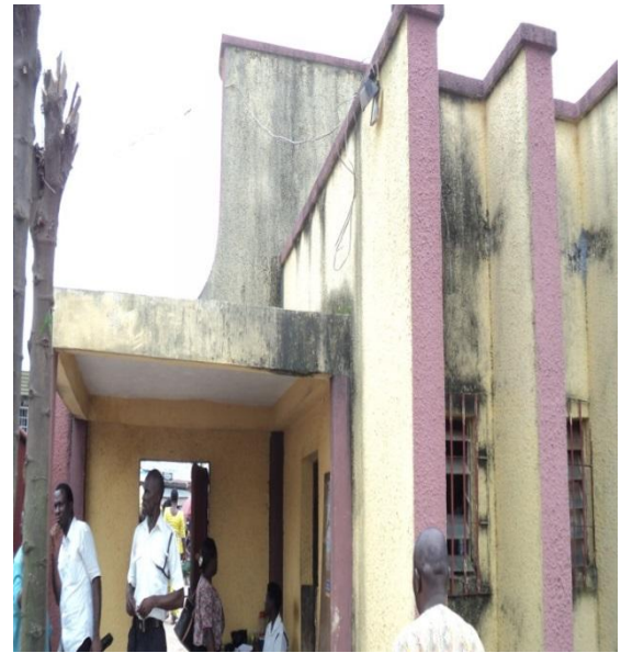
Plate 70: Stains caused by rain at external walls of the security gate house at NAUTH, Nnewi
