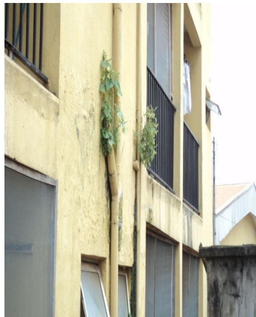
Plate 58: Plant growth at the wall/pipes of the house officers quarters at NAUTH, Nnewi.
