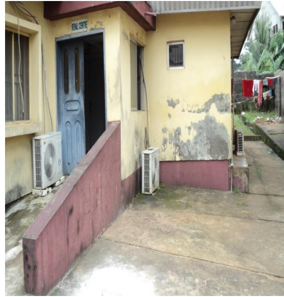
Plate 34: Detects and flaking of paint at the wall of Renal Centre, NAUTH Nnewi. Source: Researcher's field study (2017)
