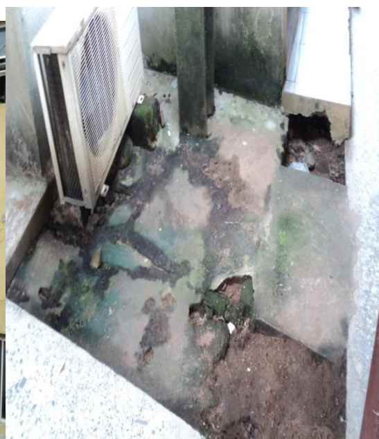
Plate 66: Dampness and Cracks at the floor Pavement of the Psychiatric building at NAUTH CHC Neni
