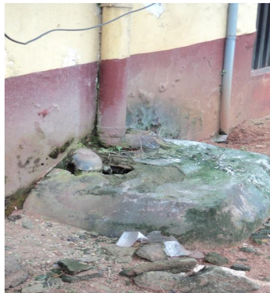
Plate 20: Showing Cracks and wall stains/defects on inspection chamber at HOQ, NAUTH Nnewi
