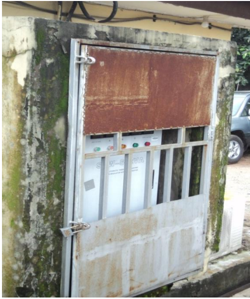
Plate 25: Efflorescence on the wall of the PCR Inverter block at Nauth, nnewi
