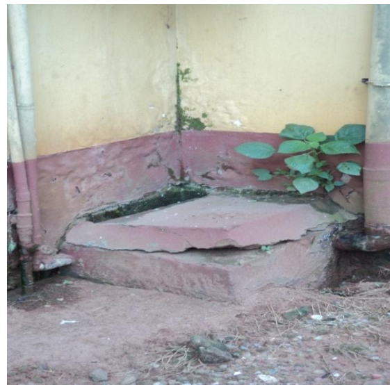
Plate 32: Plant Growth on top of Chambers at NAUTH, Nnewi.
