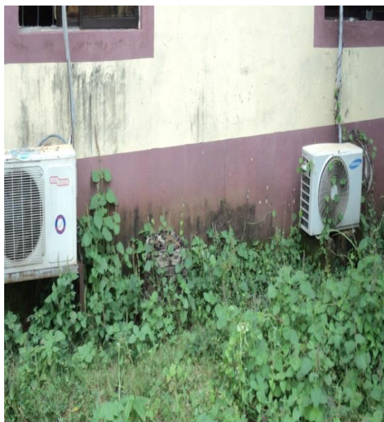
Plate 55: Stains and growth on the pipes of Air Conditioners at the back of works department at NAUTH, Nnewi.
