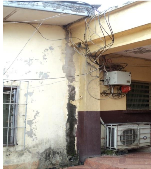
Plate 50: Dangling of electrical/Communication at the main theatre building NAUTH, Nnewi
