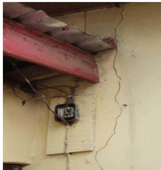
Vertical Crack at the back of the main clinic at the NAUTH, Awka outstation.
