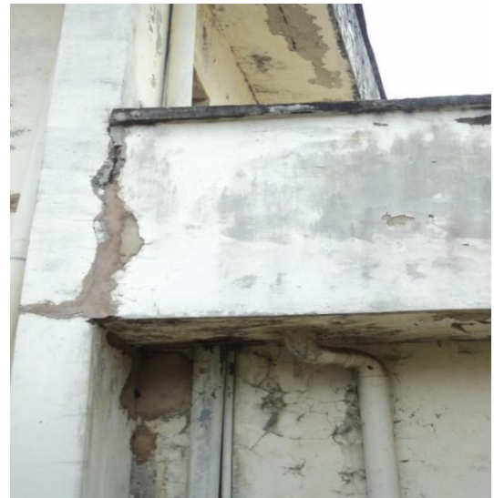
Plate 14: Crack found on the wall of the Labour Ward at NAUTH CHC Umunya Source: Researchers field study (2017)
