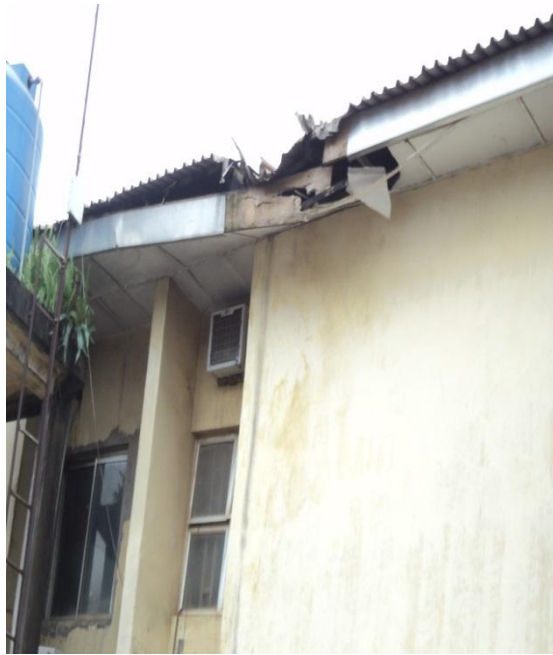
Plate 69: Damaged Aluminum roofing sheets caused by trees at the back of SON building at NAUTH, Nnewi.
