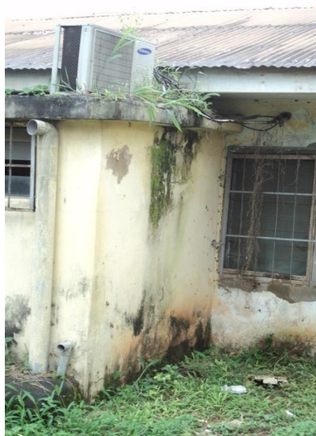
Plate 38: Plant growth on the wall and slab of the IHVN Clinical at NAUTH,Nnewi Source: Researcher's field study (2017)
