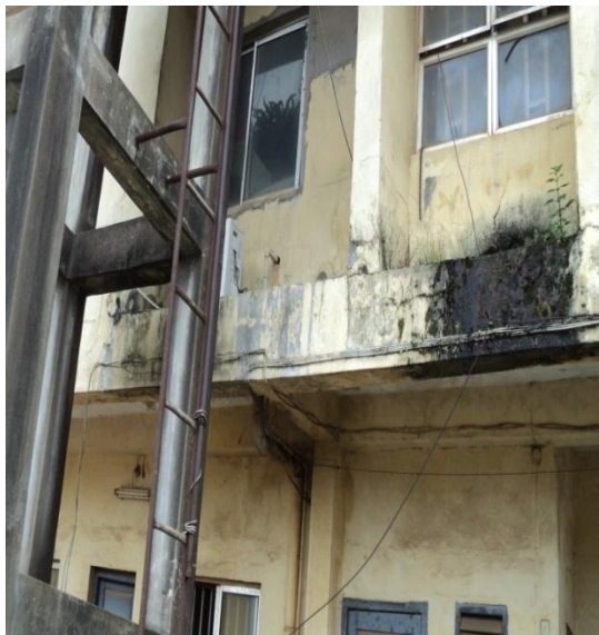
Plate 51: Dampness, Mould stains and weed Growth on the 1 st floor caused by water from Air conditioners at the Doctors call buiding at NAUTH, Nnewi
