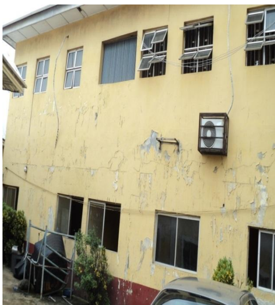
Plate 65: Flaking of paint at the external wall of the main building of the NAUTH CHC Neni.
