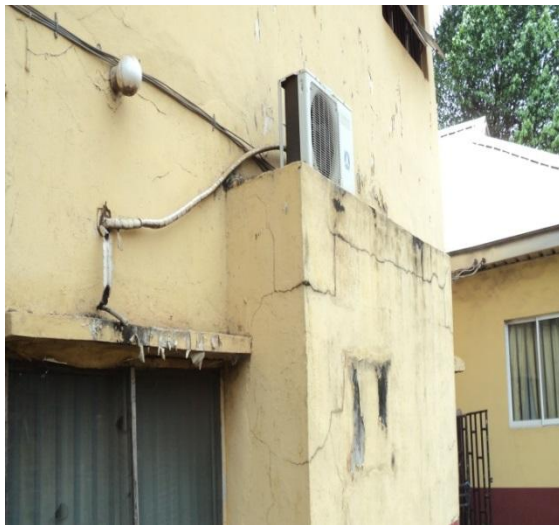
Plate 11: Crack caused by water from air condition at Radiology Building, at NAUTH
