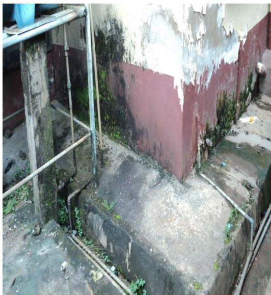
Plate 19: Defects Caused by Efflorescence on the Wall of Clinical building at NAUTH GEC Onitsha
