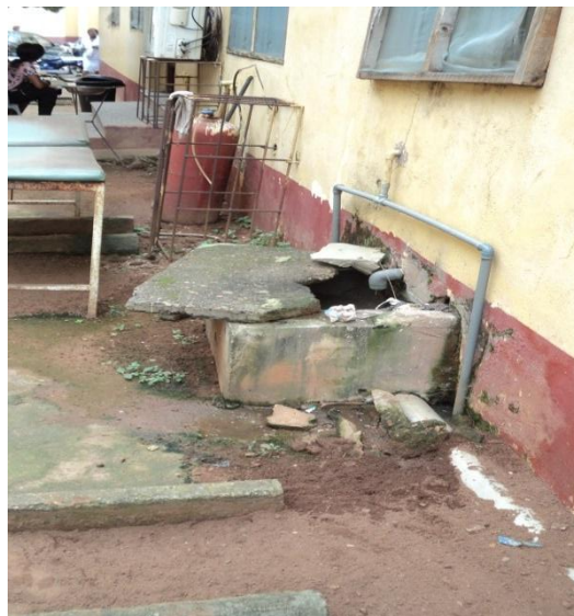
Exposed inspection Chambers at the back of the store building at NAUTH, Nnewi.
