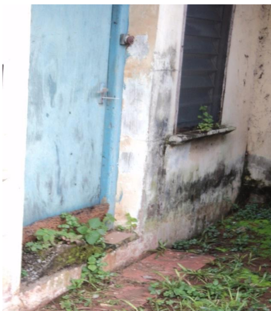
Plate 53: stains and plant growth at the window Hood of the HIV call room at NAUTH,Nnewi.
