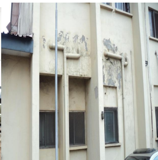
Plate 48: Peeling and Flaking of paint at the Radiology building at NAUTH,nnewi Source: Researcher's field study (2017)
