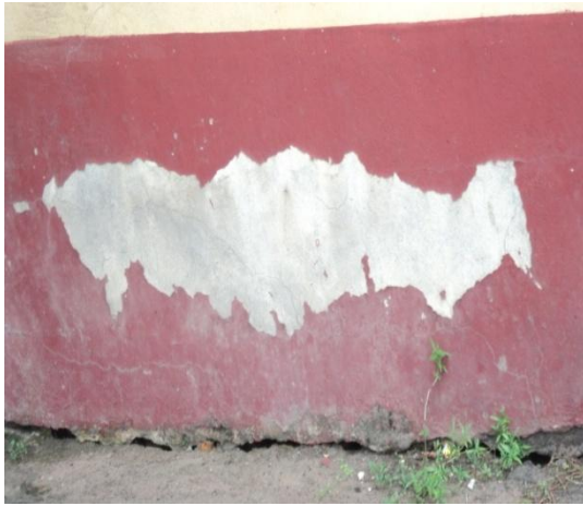
Plates 1: Longitudinal Crack and Dampness at the Foundation level of Audit extension block at Nnewi.
