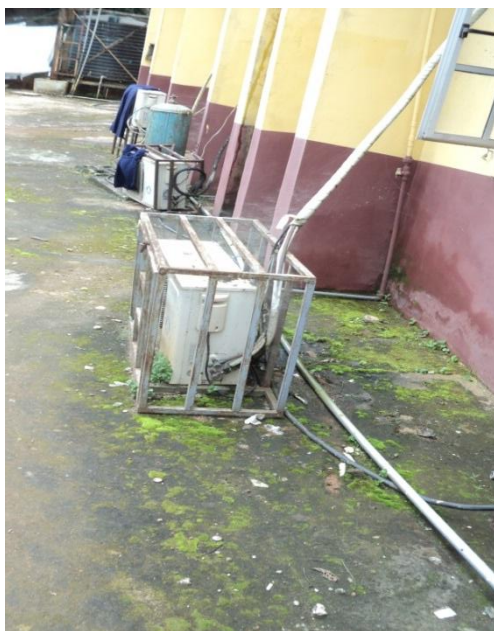
Plate 57: Efflorescences caused by dampness at the Pavement of the MOP/SOP building at NAUTH, Nnewi.
