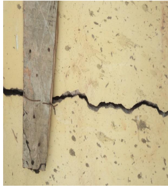
Plate 26: Bold Crack at the wall of the senior registras call building at NAUTH CHC, Umunya.
