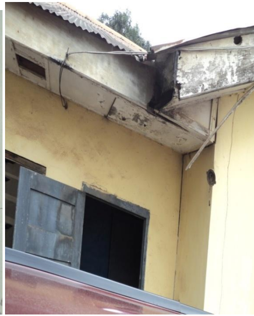
Plate 22: Vertical Crack at the joint, at Administration building at NAUTH GEC Onitsha.
