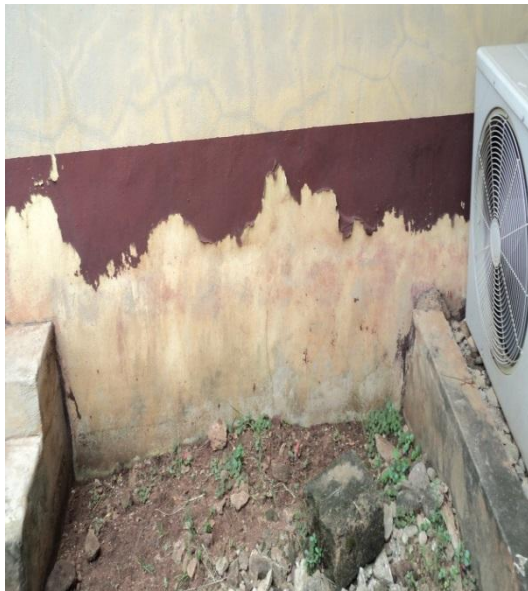
Plate 43: Horizontal cracks and flaking of Paint at the back of the security house at NAUTH CHC Ukpo. Source: Researcher's field study (2017)
