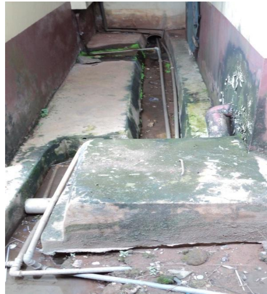
Plate 18: Crack and Mould stains on the external wall of the Laundry building, at NAUTH Nnewi
