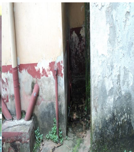
Plate 40: stains and dampness at the back of the Maternity block at NAUTH CHC Umunya Source: Researcher's field study (2017)
