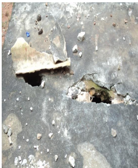
Plate 37: Broken Septic Tank/Soakaway Pit at the NAUTHGuiness Eye centre Onitsha Source: Researcher's field study (2017)
