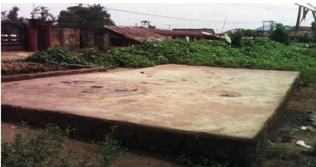
(4c) Okija pit disposal system
