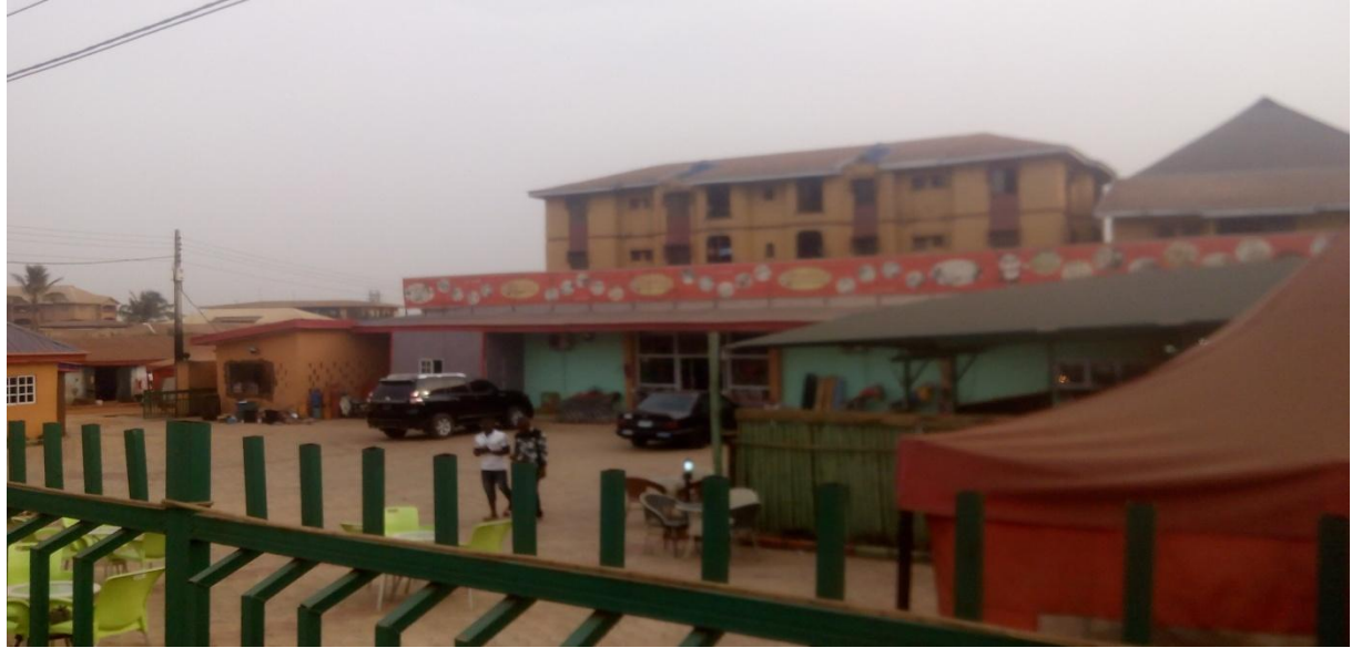
Plate 21: Njikoka Abakaliki Farmers' Multi-purpose Cooperative Society Building (Housing PANDA Restaurant and Recreation Centre), Vanco/ Ogoja Road
