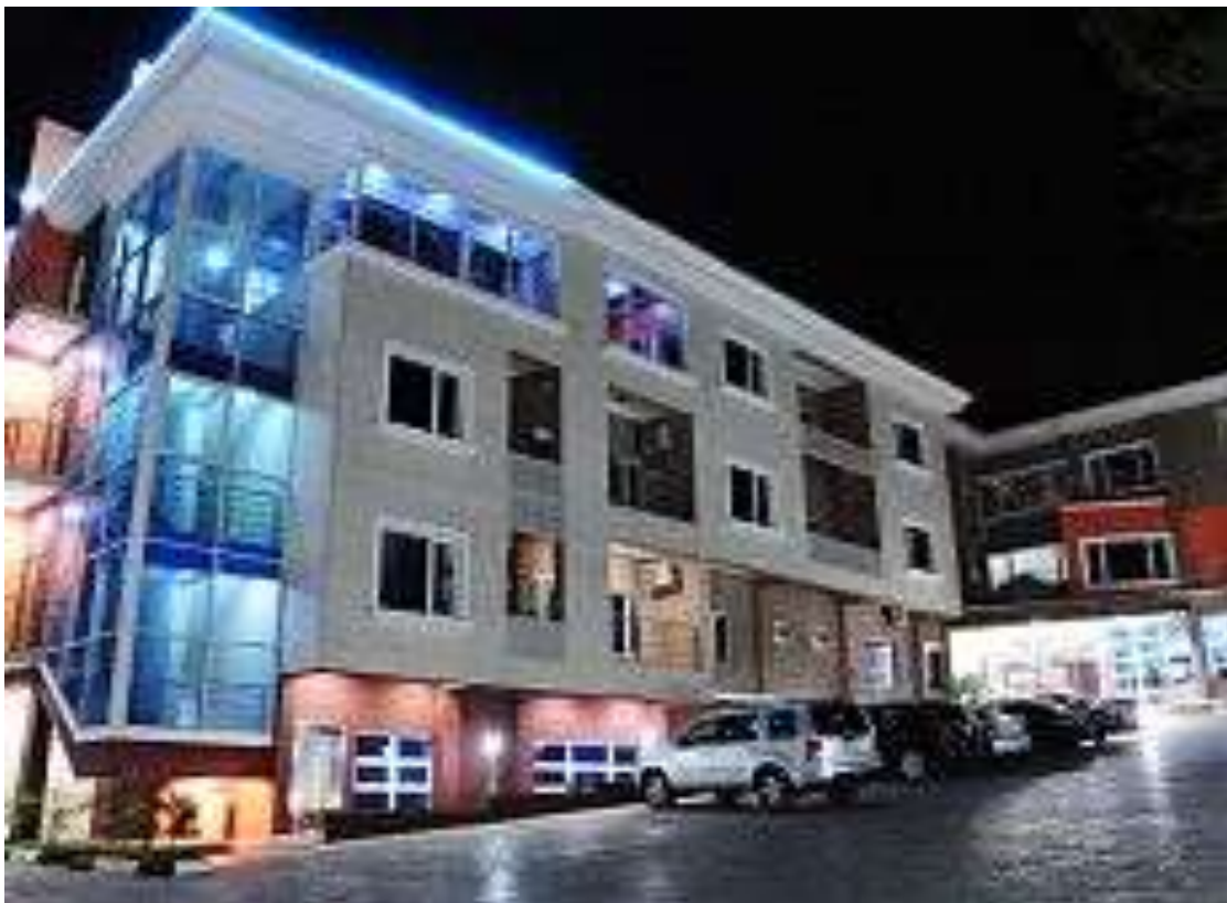
Plate 3.3: Sample of Modern Hotels with Heavy Energy Usage in Gwarinpa Housing Estate
