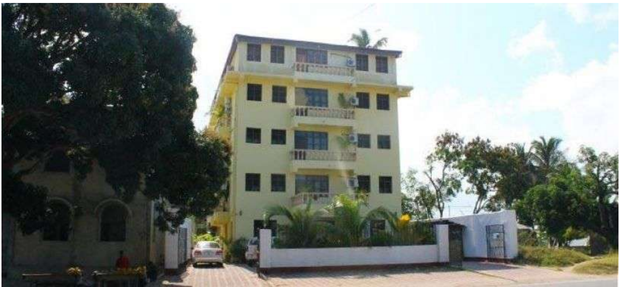
Plate3.1: Sample of Residential Building in Gwarinpa Housing Estate Source: Researchers Field Work (2016)
